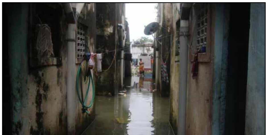
Figure 15: A flood-affected housing complex in Semmancherri Source: Chennai Floods, BBC News, 2015
