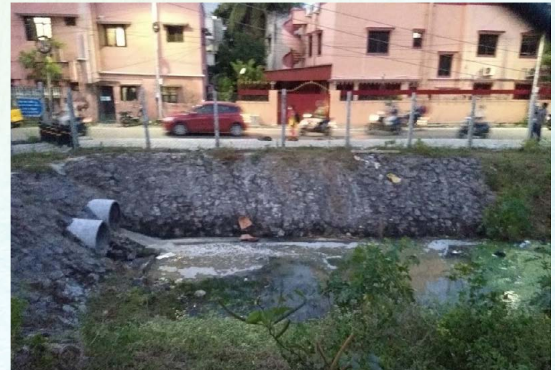
Figure 36: Sewage being let into the lake
