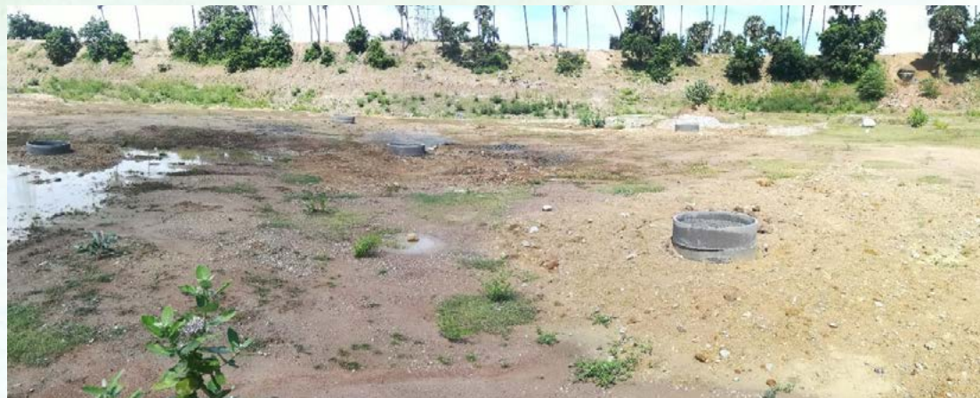
Figure 24: Recharge wells being installed in Talambur lake
