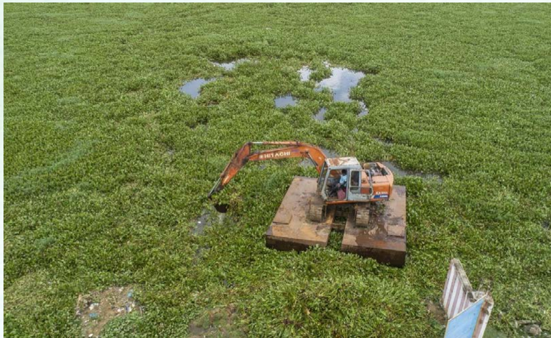
Figure 40: Aquatic weed being removed from the lake
