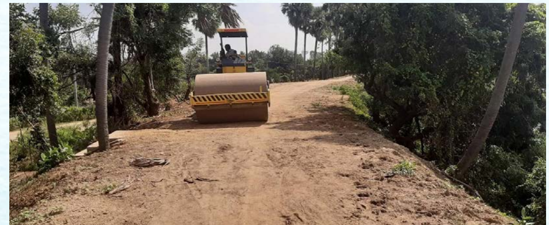
Figure 25: Bund compaction at Thalambur lake with a vibrator roller
