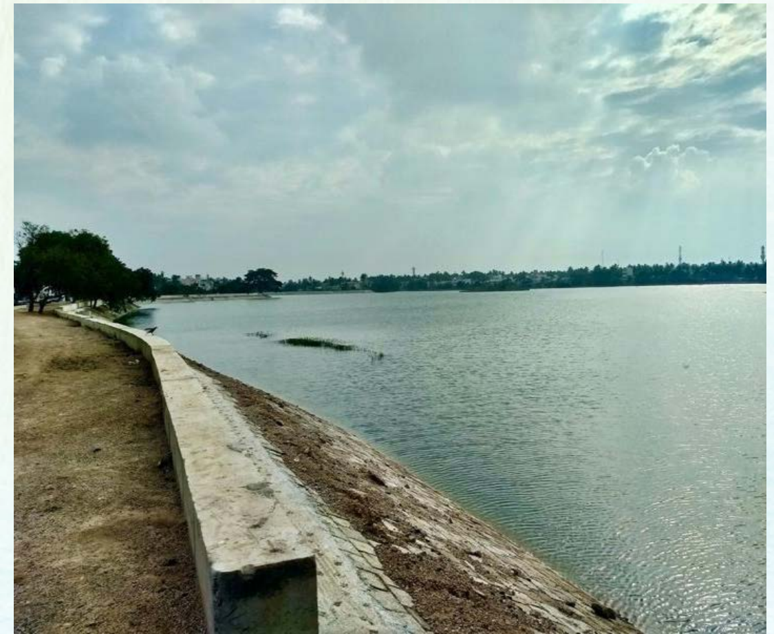
Figure 32: Concrete block acting as a bund, constructed around the lake
