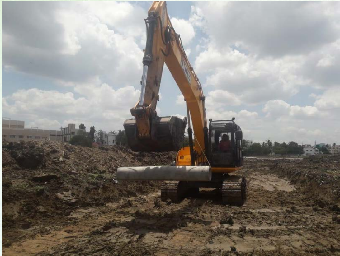
Figure 41: Silt being removed from the lake
