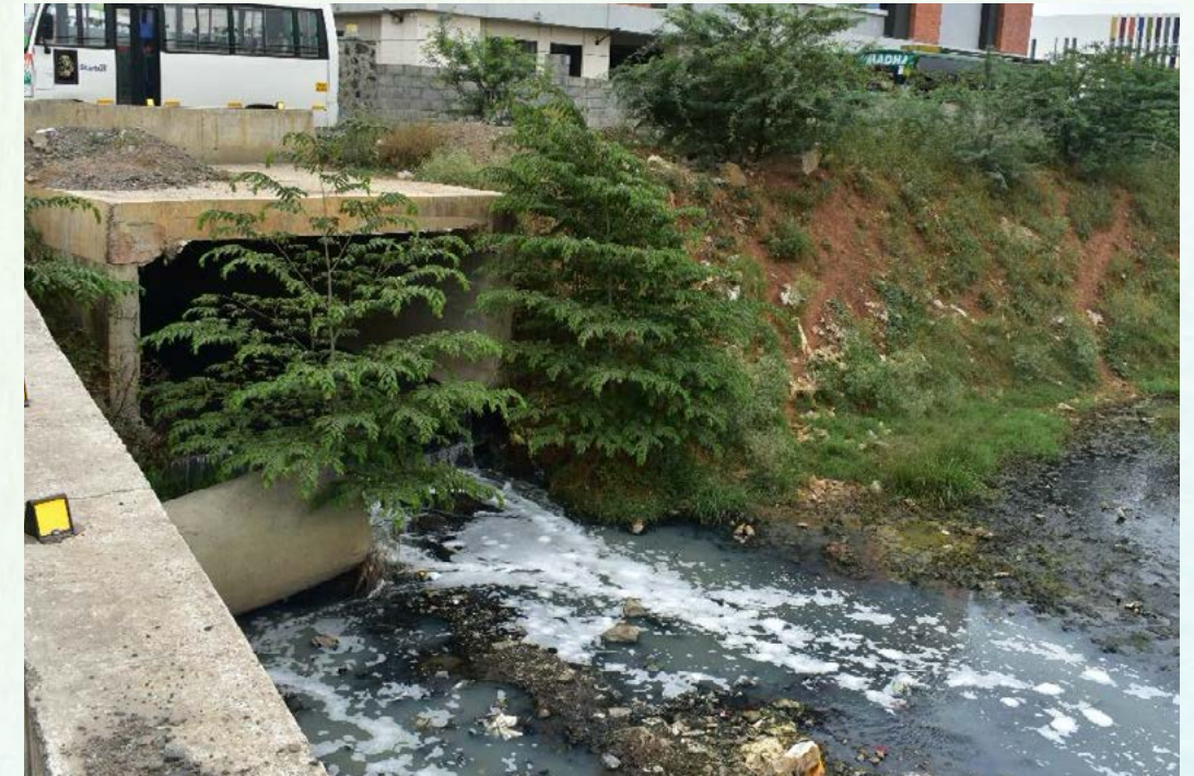
Figure 11: Sewage discharge in Pudhuthangal Lake
