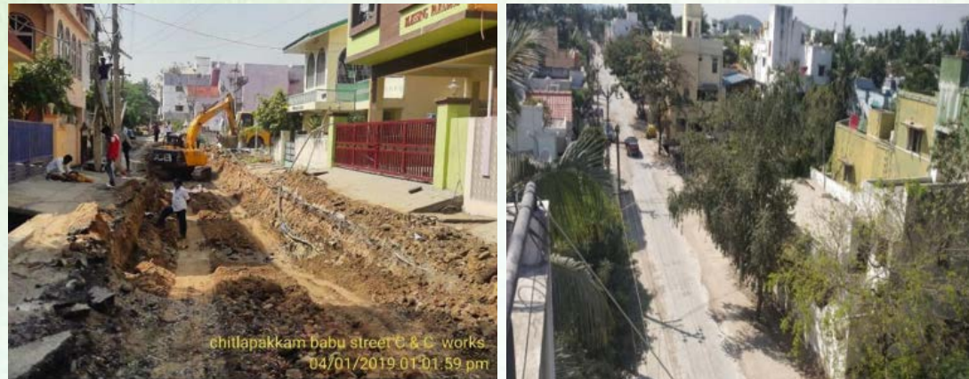
Figure 39: Cut and cover drains constructed between Chitlapakkam and Sembakkam
